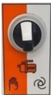
Figure 32: Selector switch pressure booster pump
