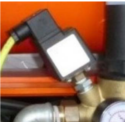
Figure 112: Pressure switch water
