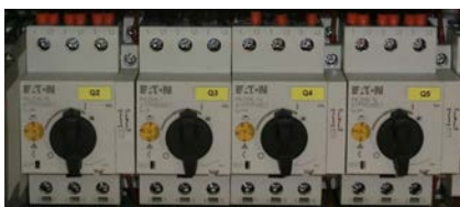
Figure 4: Motor protection switch
