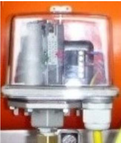
Figure 113: Pressure switch air
