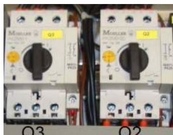
Fig. 1: Control box motor protection switch item no. 00046174
