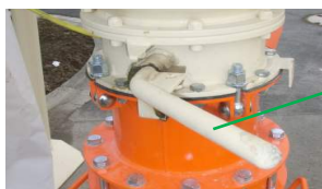
Fig. 40: Closing the silo outlet flap
