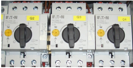
Fig. 2: Control box motor protection switch item no. 00681407
