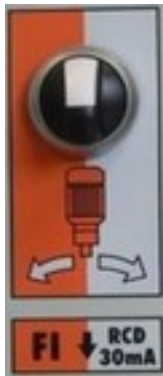
Figure 21: Pump motor selector switch
