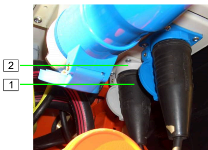
Figure 51: Connecting the vibrating unit
