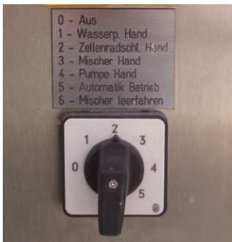
Fig. 13: Selector switch star wheel lock
