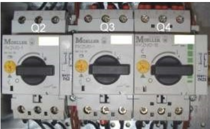
Figure 4: Motor protection switch
