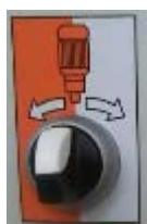
Figure 13: Pump motor selector switch
