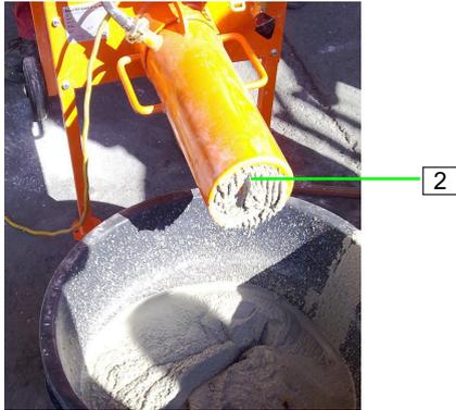
2. Check mortar consistency at the mortar outlet (2).
