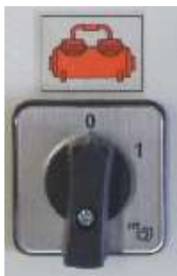
Figure 22: Air compressor selector switch
