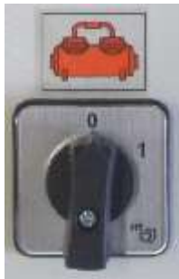
Figure 18: Air compressor selector switch
