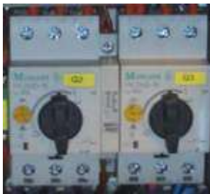
Figure 5: Motor protection switch
