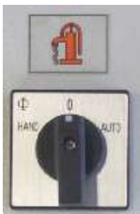
Figure 19: Selector switch pressure booster pump
