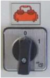
Figure 20: Air compressor selector switch
