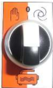
Figure 19: Selector switch pressure booster pump
