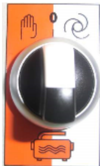
Figure 19: Selector switch pressure booster pump
