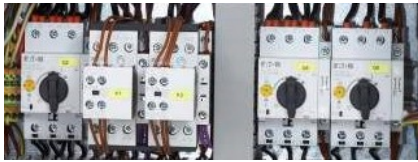
Figure 4: Motor protection switch
