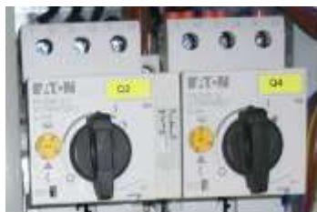
Figure 4: Motor protection switch
