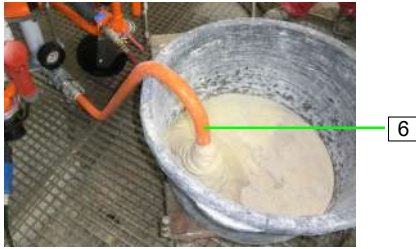
Figure 59: Checking the consistency
