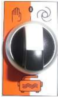
Figure 21: Selector switch pressure booster pump
