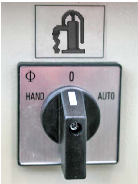
Fig. 14: Water pump – operation modes
