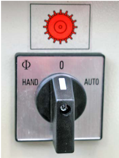
Fig. 13: Cellular wheel – operation modes
