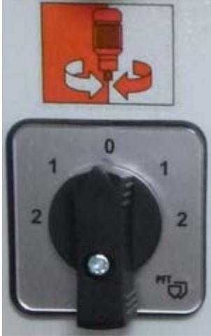
Figure 15: Pump motor selector switch
