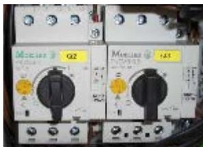
Figure 4: Motor protection switch
