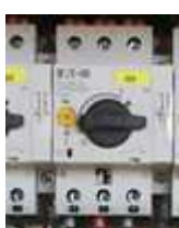
Fig. 22: Check the motor protection switch
