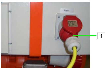
Abb. 26: Stromanschlüsse
